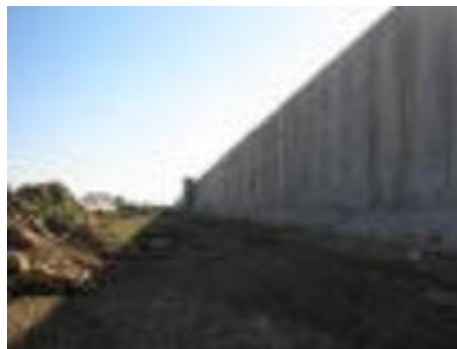
The security wall surrounding Qalqilya
